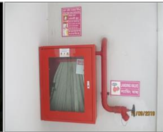
External photo(s) of the production unit(s) Fire hosepipe.JPG
