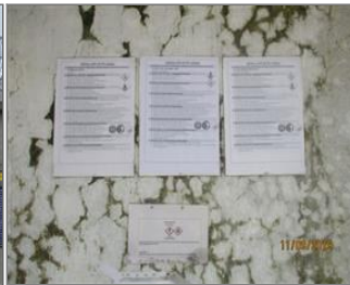
External photo(s) of the production unit(s) MSDS posted in the local language.JPG
