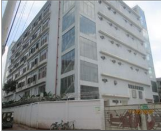
External photo(s) of the production unit(s) Factory building.JPG
